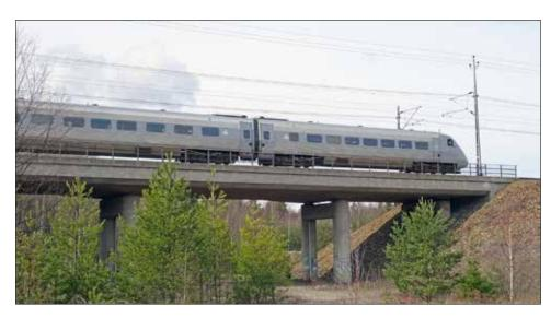
A three span concrete railway bridge in Södertälje, Pershagen.
